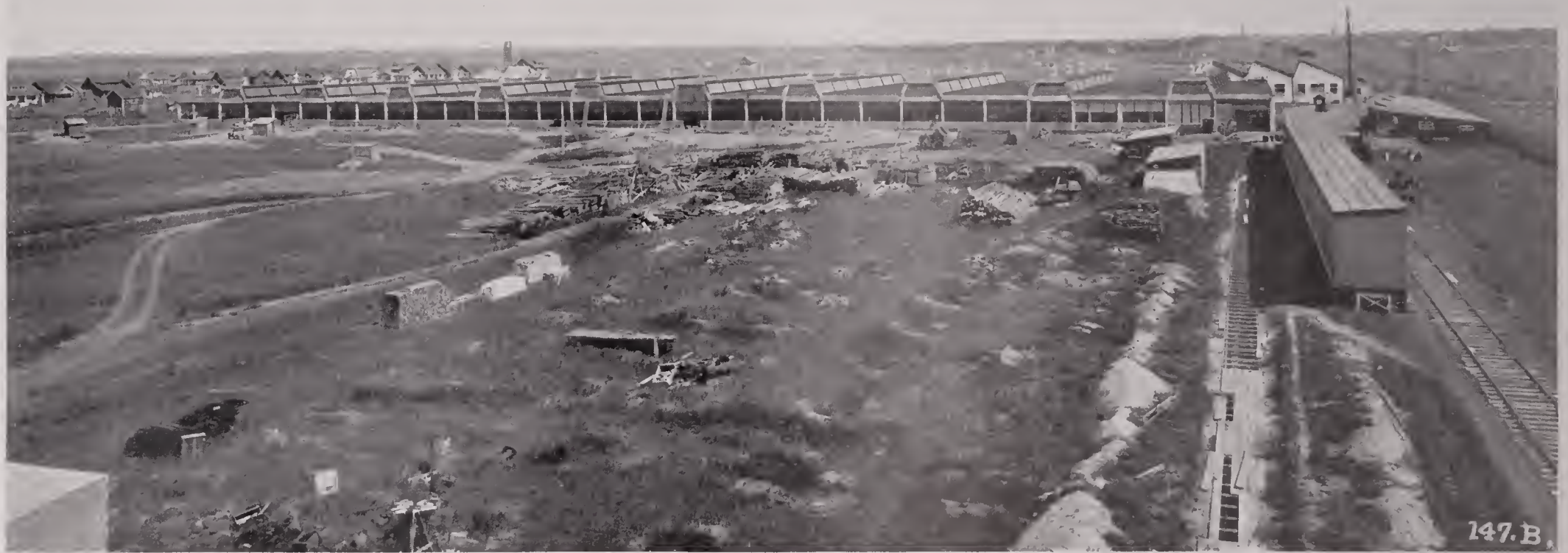
VIEW OF MAIN PRODUCTION UNIT FROM POWER HOUSE
